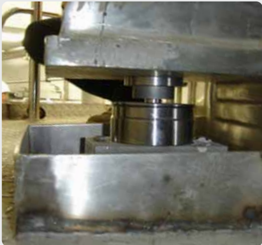
▲ Installation of compression load cells under vessels with brackets
